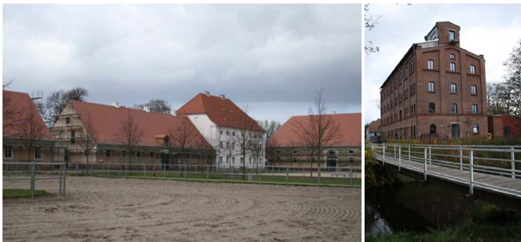
Neustadt-Dosse: scaffolding at some of the “Hauptgestüt”-building
